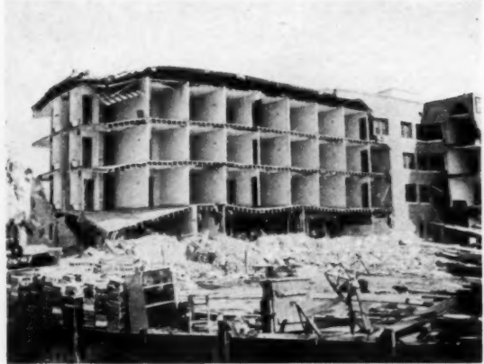
FIG. 9. CALIFORNIAN HOTEL, SHOWING ENTIRE DESTRUCTION OF BRICK RETAINING WALL
